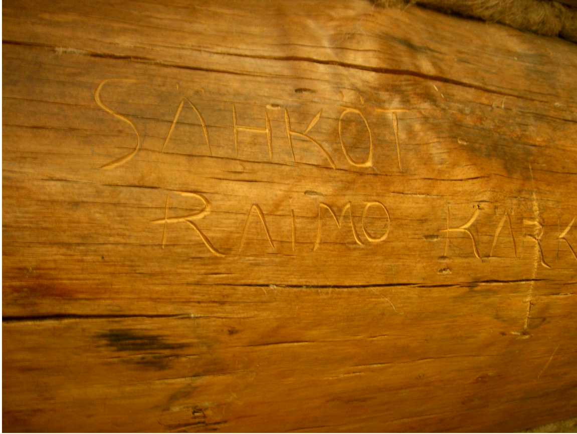
Figure 1767. Rynnänen's tribute to the church's lighting engineer.
