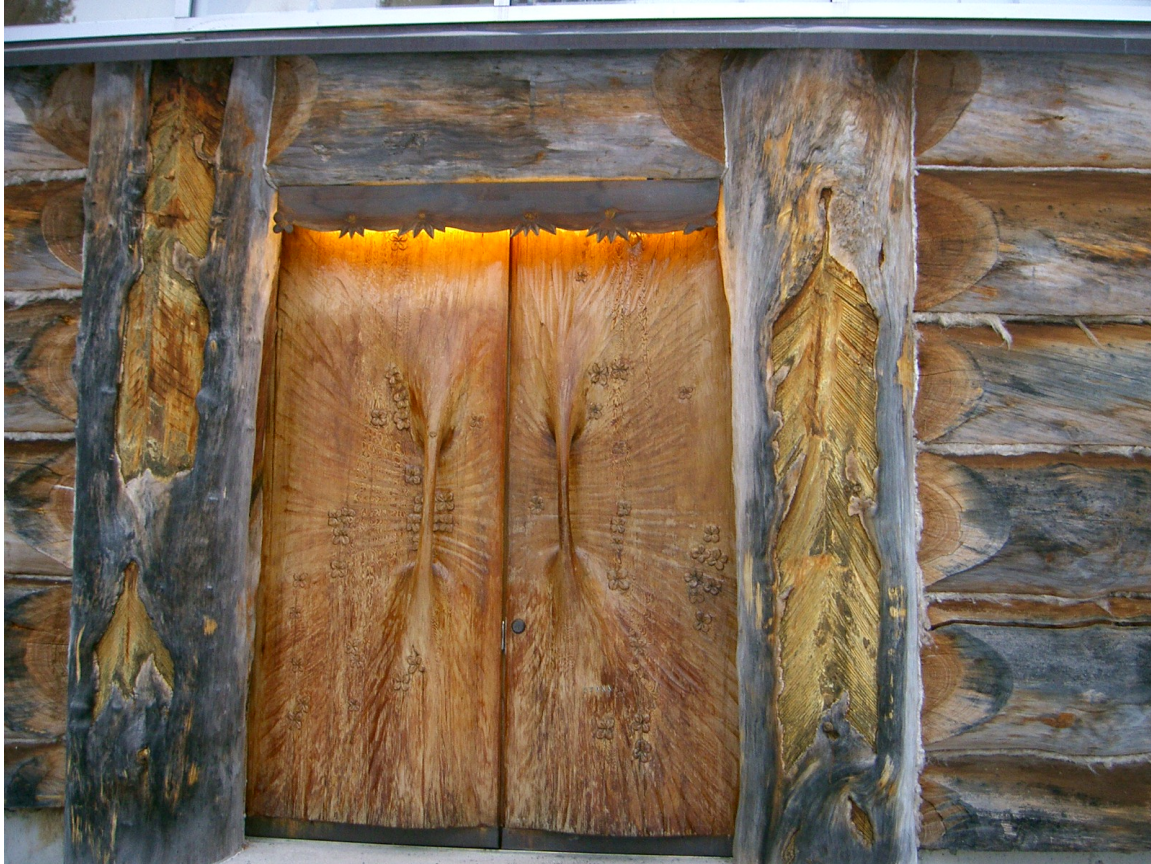
Figure 1748. Front door framed by upright beams, the latter showing sapping striations from the period when they were newly cut.
