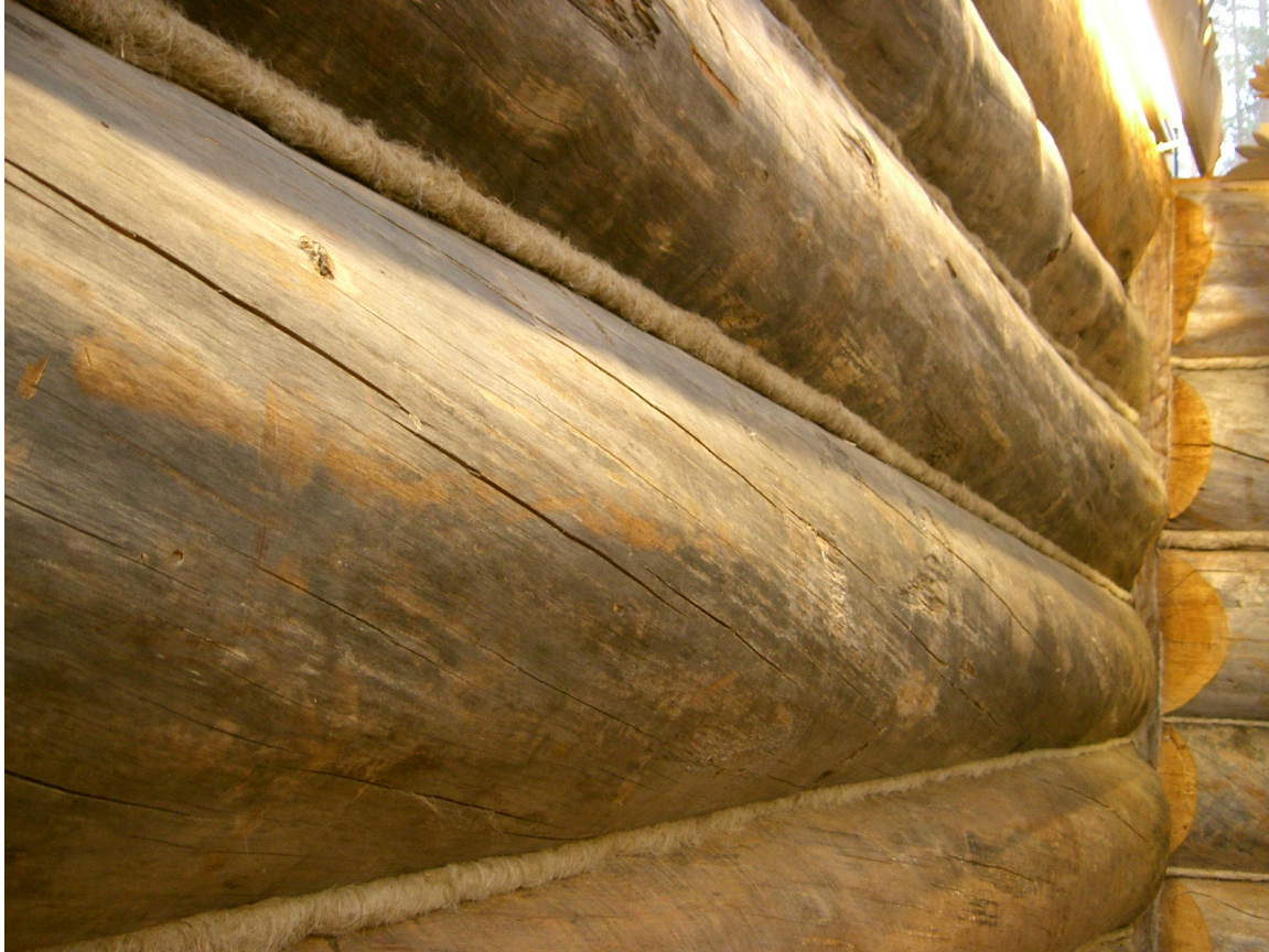
Figure 1762. Church wall showing logs and fiber chinking.
