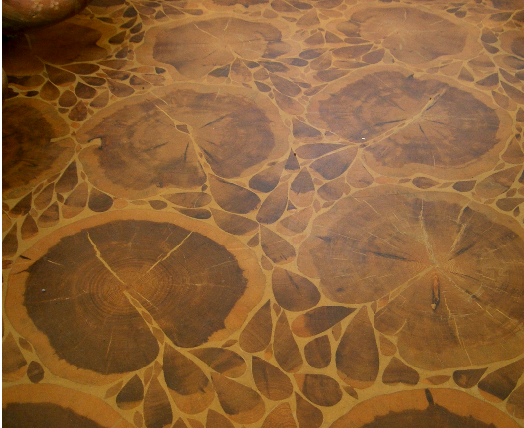
Figure 1753. Flooring, showing pine trunks, tear-shaped pieces, and surrounding mastik.
